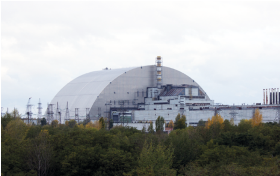
1. The containment shell of the damaged No. 4 reactor at the Chernobyl nuclear power plant in Ukraine and its first sarcophagus, due to come into service in 2019. 108 m high, 162 m wide and with a span of 257 m, it is designed to last 100 years.
