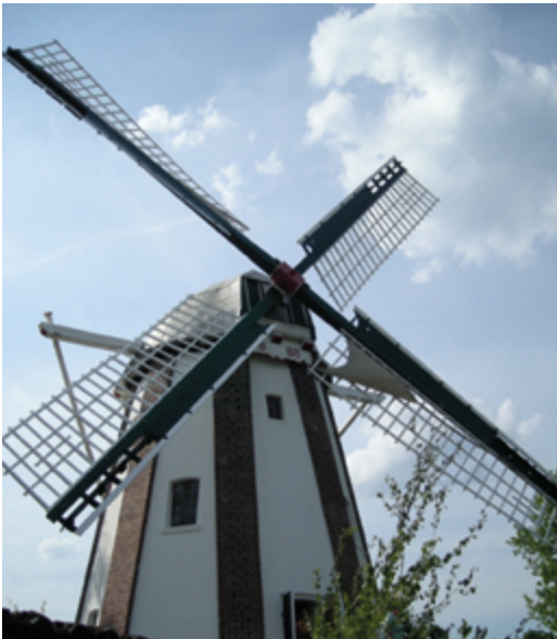
Windmill from the XIX e century in northern Germany. Note the twisting of the rotor blades.
